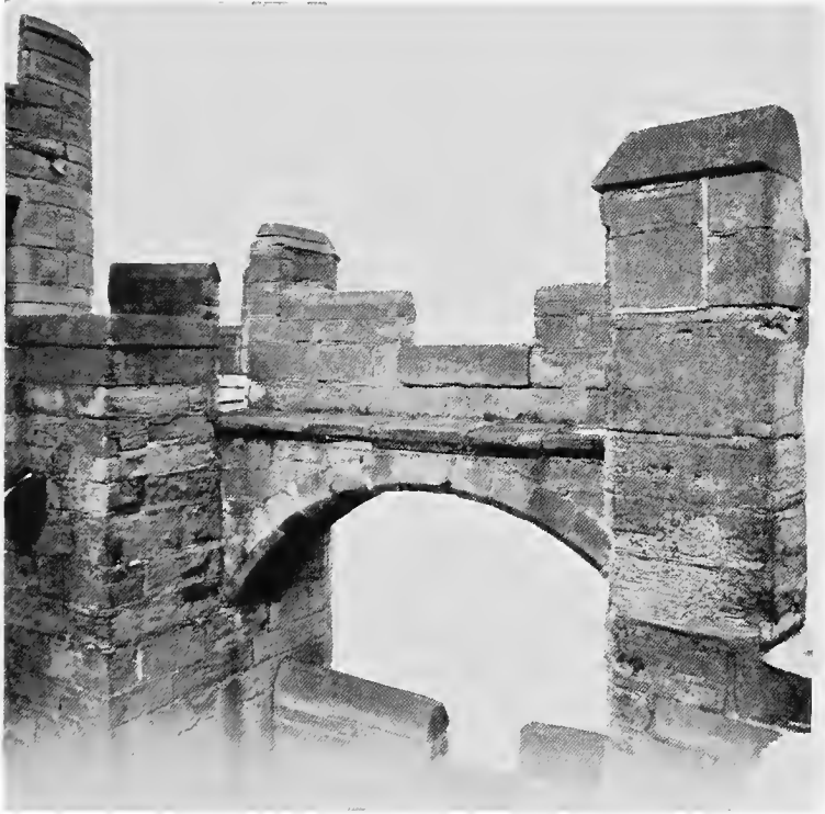
AN ARCH OF THE CLOCK TOWER, WARWICK CASTLE.
